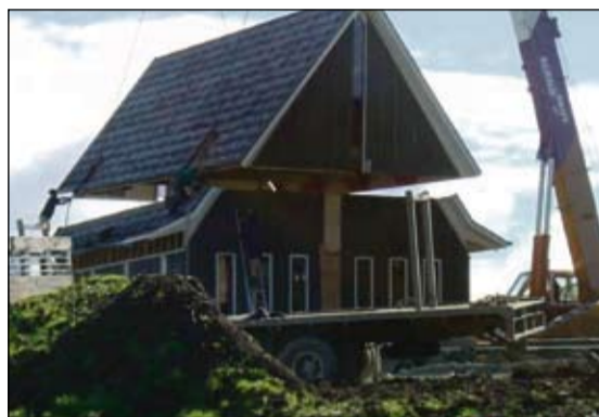
Cranes lower the church into place
